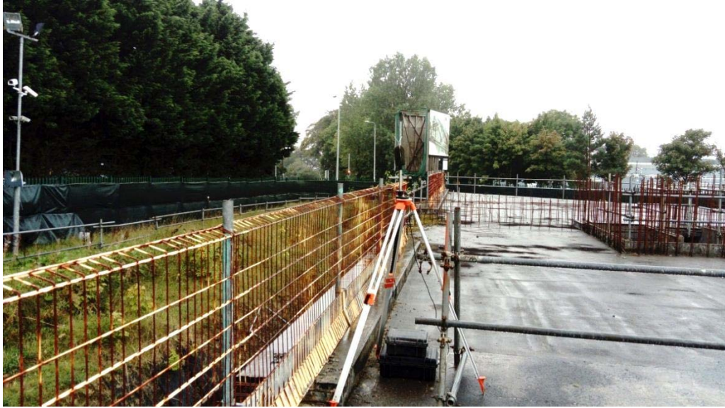
Photograph 9.2 N2, looking SW towards site corner.
