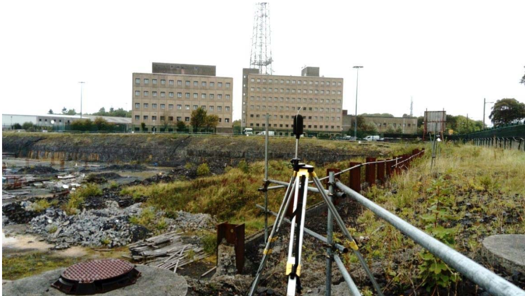
Photograph 9.3 N3, looking NE towards Eir site.
